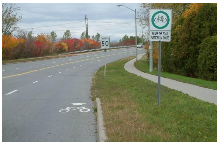
Figure 6.6 – Wide Curb Lane with Bicycle Pavement Markings and Signing (City of Ottawa)
