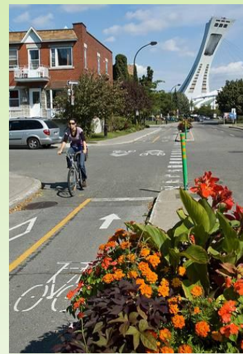
Figure 6.12 – Example of a Two-way Cycle Track in Montreal, Quebec
