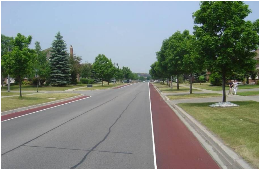
Figure 6.27 Microsurfacing – Town of Richmond Hill, ON
