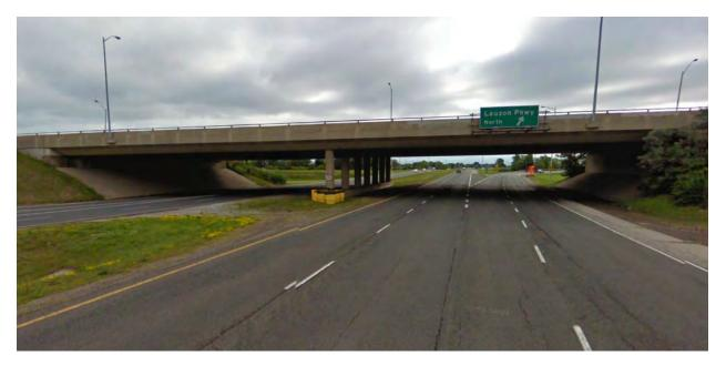
The Lauzon Parkway Bridge over the CP Rail is a 3-span pre-stressed concrete girder bridge built in 1980. It has a total span length and width of approximately 61.9 m and 24.6 m respectively. The structure was rehabilitated in 2008. Work on the structure included converting the existing abutments to semi-integral abutments and constructing new approach slabs. The structure is illustrated in Exhibit [A.4-11.
